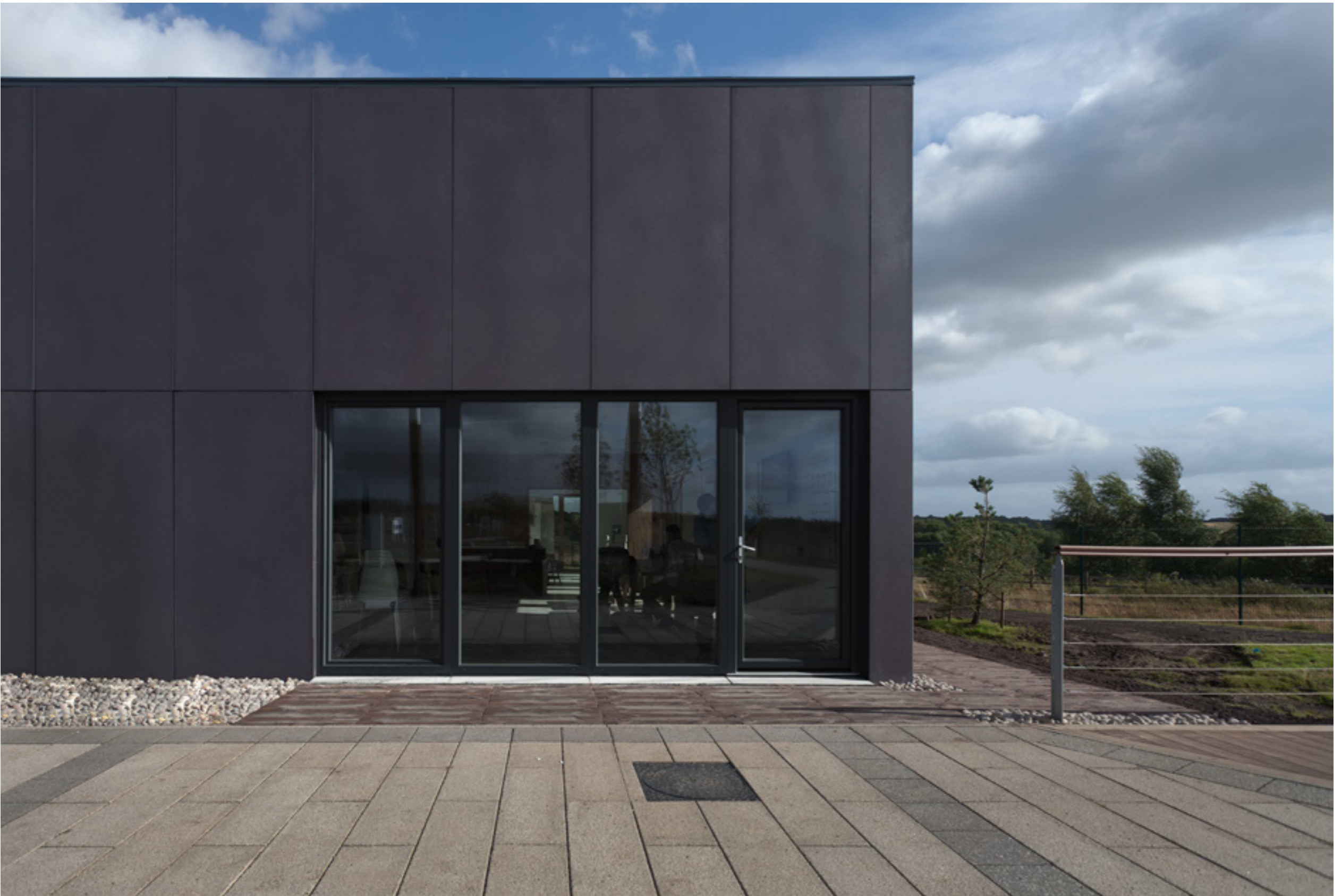
BRE Innovation Centre, Ravenscraig for Kraft Architecture
